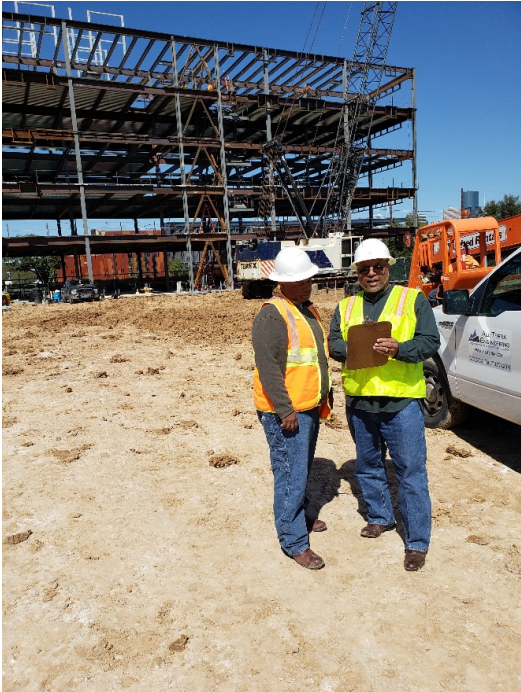
Construction Manager Zack Martin, on right, confers with inspector Darron Thompson (03/02/20)
